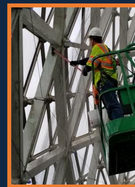
Corrosion Potential Testing
